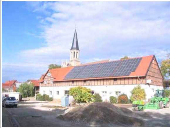
More solar farm power in Dardesheim. Photo by Ziggy Kleinau
