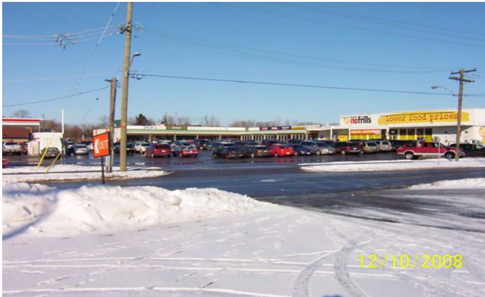
Mid-Town Mall: Example of Potential Greyfield Development Site
